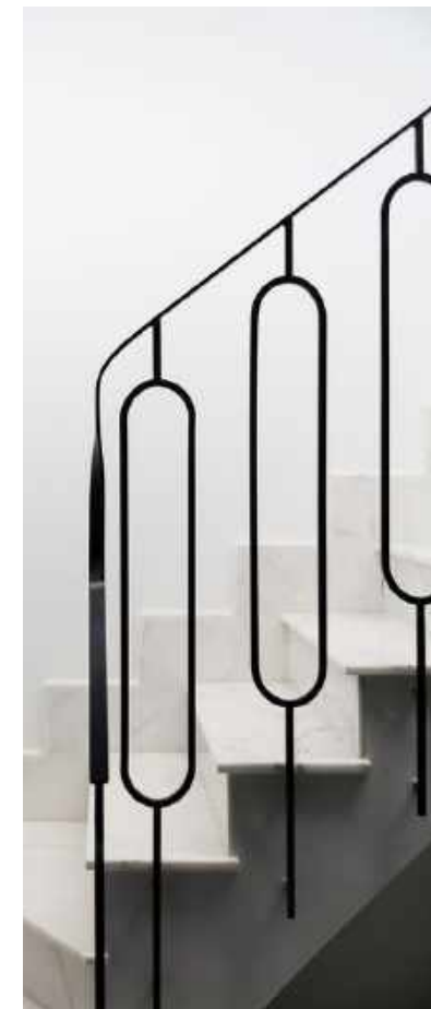
Balustrade fixed to the side of each tread
