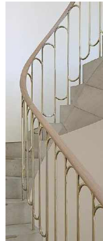
Balustrade fixed to the top of each tread
